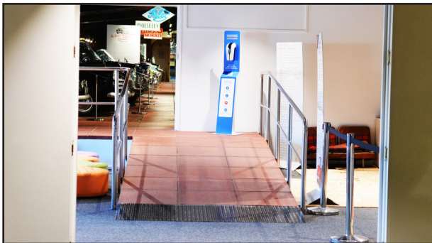
Family Room ramp
